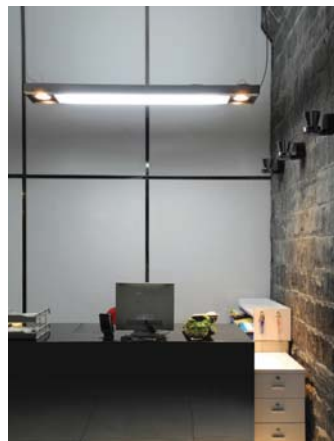
Ceiling base for power supply and suspension wire
